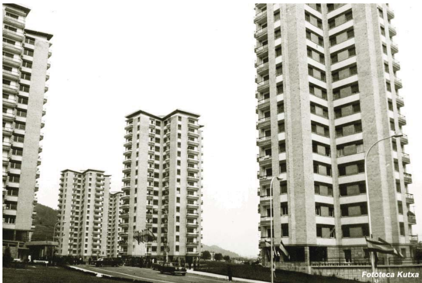
Figure 3: Photograph of the Bidebieta Towers.
